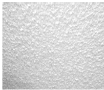
Trowelled on asbestos
