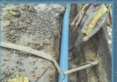
Van Cleef was contracted by the borough of Island heights to provide design, bidding and construction services for the installation of an 8" diameter C900 PVC water main extension along Lake Drive. In general, the work will include furnishing of all labor, materials and equipment necessary to complete the replacement (relocation) and abandonment of the Borough's existing 4" ACP and Cast Iron water main along Lake Drive, as shown on the Drawings and as described in the Specifications.
